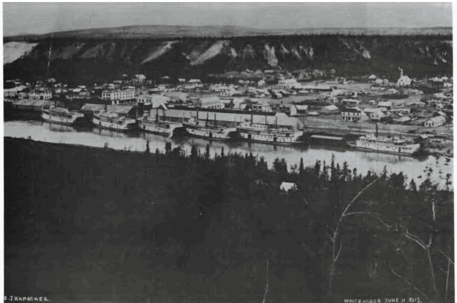
Figure 1. Whitehorse - June 11, 1913. Note "bridle path" on face of escarpment. (Photo taken by E.J. Hamacher; original print loaned by W.D. McBride, Whitehorse.)
