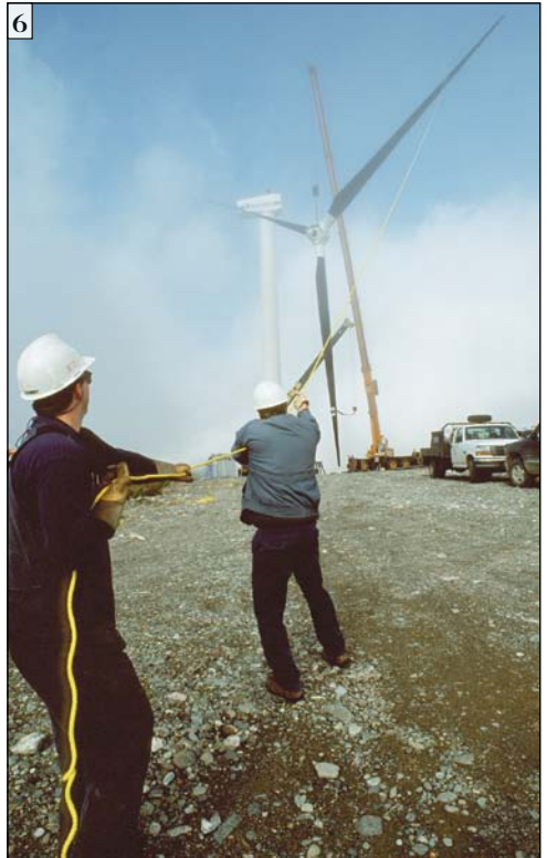
1) Tightening one of the many bolts holding the tower in place. 2) Joining a blade to the hub. 3) Looking up the ladder, inside the tower. 4, 6, 7) Mounting the blade/hub assembly to the nacelle. 5) Lining up the second part of the tower.
