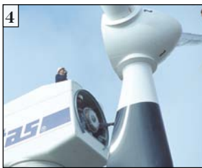
1) Tightening one of the many bolts holding the tower in place. 2) Joining a blade to the hub. 3) Looking up the ladder, inside the tower. 4, 6, 7) Mounting the blade/hub assembly to the nacelle. 5) Lining up the second part of the tower.
